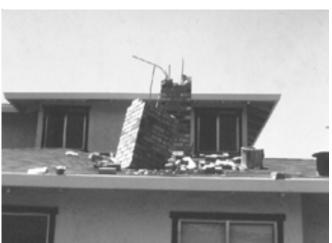
Figure 34 - Morgan Hill Earthquake. Broken chimney fell on roof
