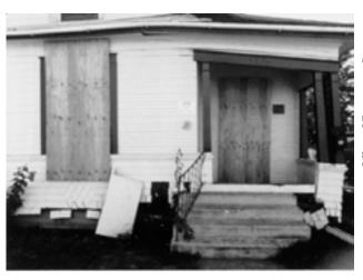
**Figure 13** - This home wasn't bolted and slid off its foundation. Sometimes the damage can be so bad that houses have to be demolished.
