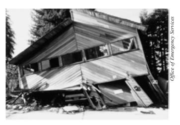
**Figure 29** - This mountain home was built over a garage, and its walls were not strong enough to withstand an earthquake.
