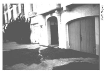
**Figure 40** - Loma Prieta Earthquake, October 17, 1989. Lateral spreading, liquefaction and sand boils caused extensive damage in the Marina District of San Francisco, about 60 miles away from the epicenter.
