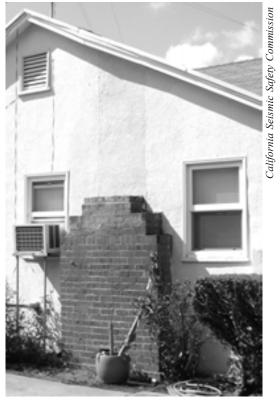
**Figure 35** - Photo showing damaged chimney removed. Note that the fireplace is now not functional.
