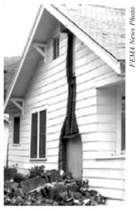
**Figure 4 - Northridge Earthquake, Jan. 17, 1994** Chimney Collapse - common type of damage to unreinforced masonry.
