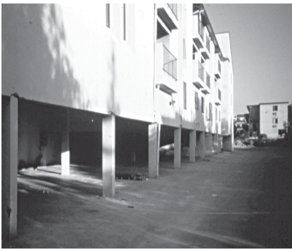
Figure 30 —Apartments with tuck-under parking like this can collapse. This building is leaning but did not collapse in the 1994 Northridge earthquake.
