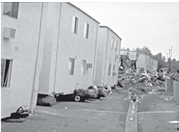
Figure 31 —A similar apartment building's soft story collapsed on cars during the same earthquake.
