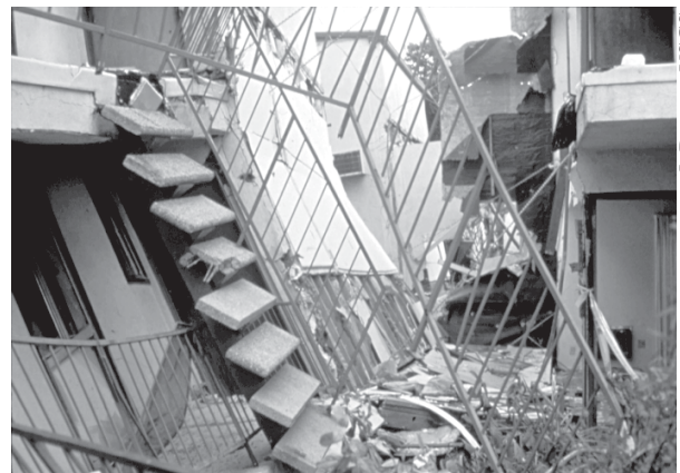
Figure 36 - Stairs to an apartment building collapsed during the 1994 Northridge earthquake.
