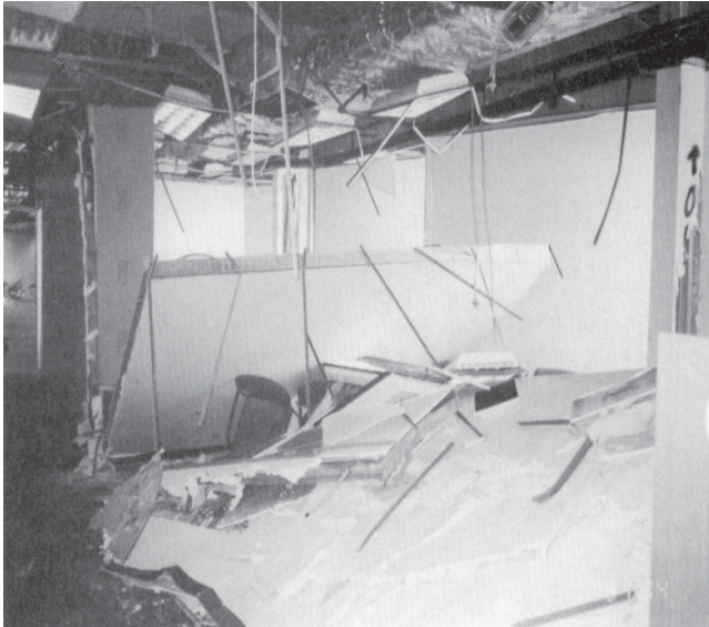
Figure 60 - Partitions and ceilings toppled onto office spaces during the 1994 Northridge Earthquake.
