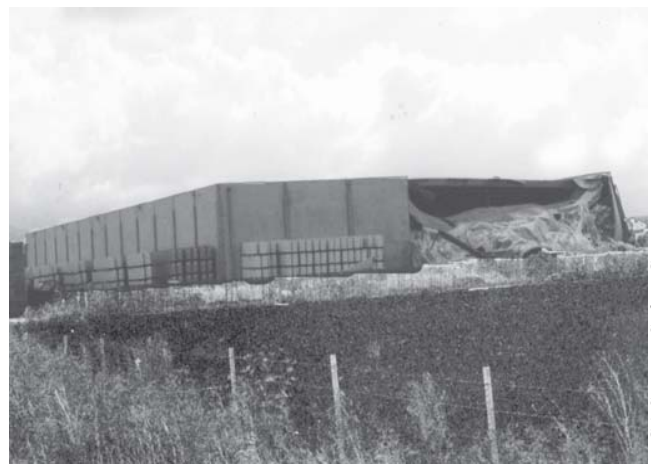
Figure 41 - Pallets of canned goods stored in this building fell off the shelves during the 1989 Loma Prieta earthquake and pushed out the concrete wall of this Hollister warehouse.
