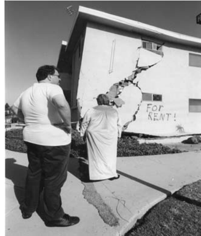
Figure 2 - Northridge Earthquake, Jan. 17, 1994. Collapse of the lower, soft story of this apartment rendered it uninhabitable.
