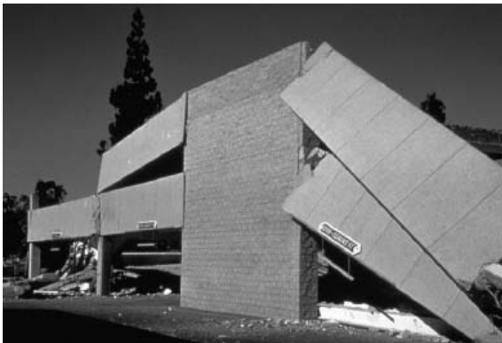
Figure 5 - Concrete Parking Structure Collapse.
