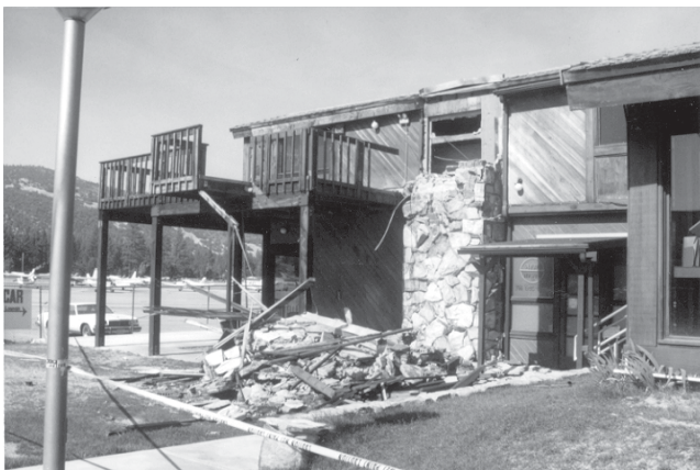
Figure 35 - The chimney on this building fell on the stair-way in the 1992 Big Bear earthquake, cutting off a means of escape for persons on the second floor.
