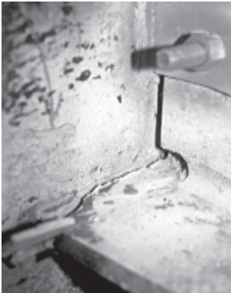
Figure 27 —This steel frame connection unexpectedly cracked in the 1994 Northridge earthquake.
