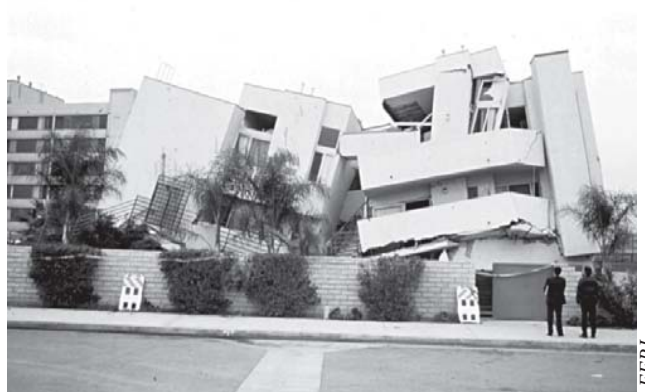
Figure 32 —This modern wood-frame apartment building had a central driveway. It collapsed inward over unbraced entrances to crush first-story parking during the 1994 Northridge earthquake.
