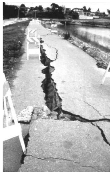
Figure 67 - Lateral Spreading. Loma Prieta Earthquake, October 17, 1989. Lateral spreading damage levee road along the San Lorenzo River.
