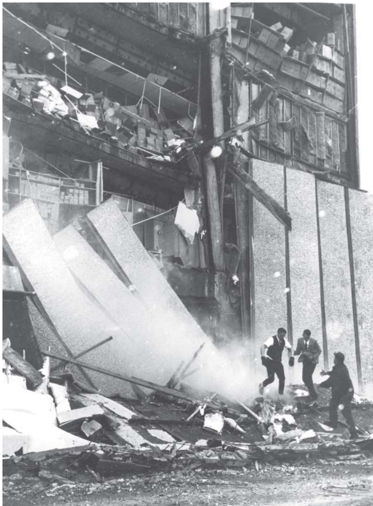
Figure 37 - Cladding on this store in Anchorage failed in the 1964 Alaska earthquake.
