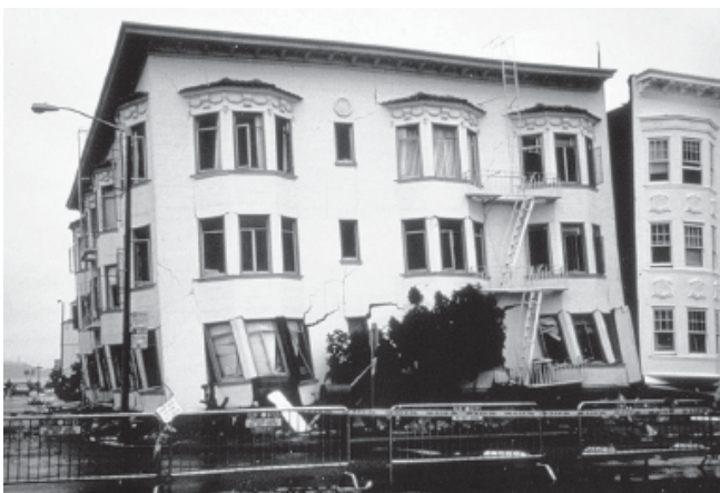
Figure 68 - Liquefaction caused differential settlement under this building and increased damage during the Loma Prieta Earthquake.
