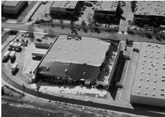
Figure 1 - Partial Collapse of an Industrial Building. Poor connections between the walls and the roof caused this collapse.
