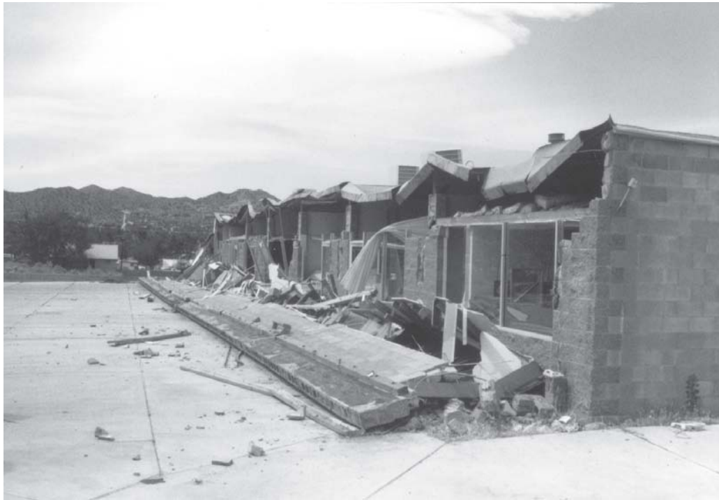
Figure 15 — Wall Anchors Can Prevent Failures Like This. Even newer buildings are not immune to earthquakes. This reinforced masonry strip mall was built in the 1980's but did not comply with the building code. The wall anchorage failed in the 1992 Landers Earthquake. Its front wall fell into the parking lot.
