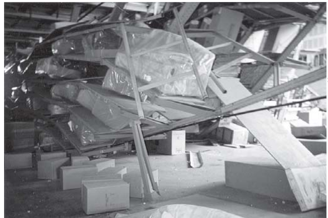
Figure 42 - The storage rack collapsed in this warehouse-style retail store during the 1994 Northridge earthquake. Heavy items such as the sofa in the center of the photo crashed to the ground and could have injured employees and shoppers.
