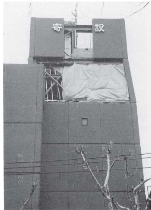
Figure 29 —A six-story steel braced frame building was damaged after the 1995 Kobe Earthquake in Japan. 4,000 to 8,000 small commercial buildings and 1,000 to 2,000 large commercial buildings were destroyed or severely damaged in that event.
