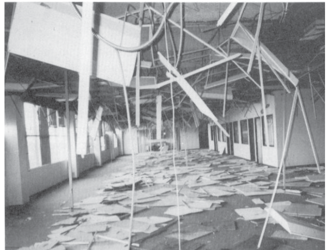
Figure 53 - This building sustained extensive interior nonstructural damage during the 1994 Northridge earthquake. Parts of the ceiling grid and tiles have fallen.
