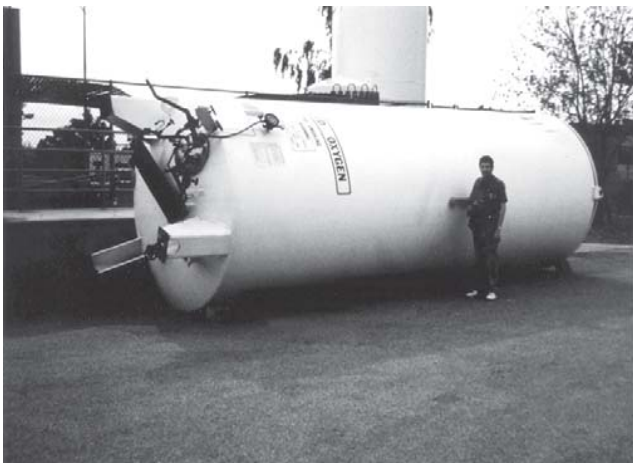
Figure 46 - The support pedestal system of this oxygen tank at Olive View Medical Center was damaged after the 1994 Northridge earthquake, leaving the tank leaning. The tank is shown after it was removed to allow for installation of a replacement unit.
