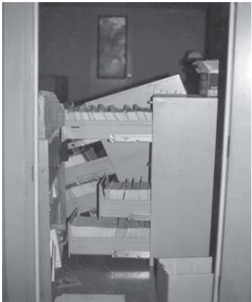
Figure 3 - File cabinet drawers can slide open and unbolted cabinets can topple during earthquakes.
