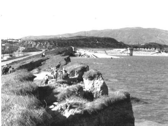
Figure 69 - Lower San Fernando Dam that was badly damaged by the 1971 San Fernando Earthquake.
