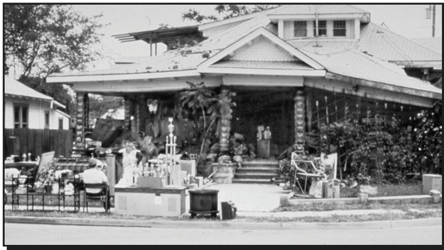
Damage from magnitude 6.7 earthquake
