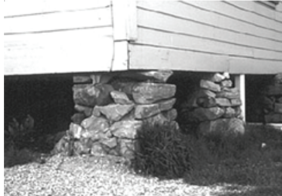
Figure 19 - This is an unreinforced stone foundation. They typically fail during earthquakes.
