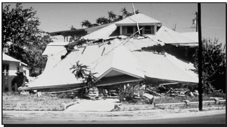
Additional damage from aftershocks
